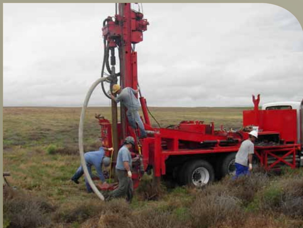
Development of a new groundwater monitoring well
